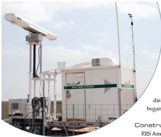
Pattern Energy has installed MERLIN SCADA radar technology for real-time bird mortality risk mitigation.
