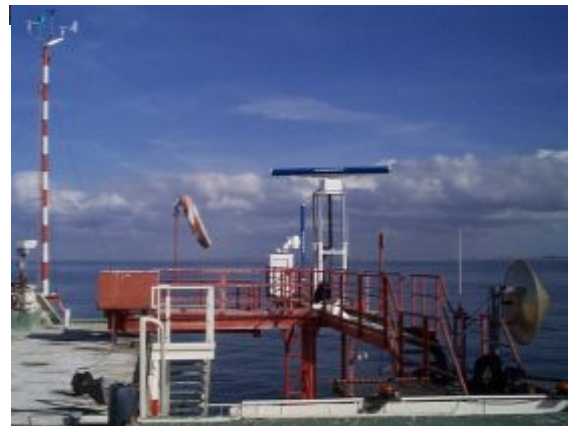
MERLIN XS2530f fixed installation on offshore research platform in the North Sea off the Dutch coast (2003) used to collect 2 years of bird data for siting of offshore the Norzeewind wind farm.
