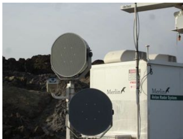
LRAD bioacoustic deterrent units installed onto the master MERLIN radar unit trailer and positions to cover control zones. Note: a DeTect laser deterrent unit (LDU) is also mounted on the support stand.
