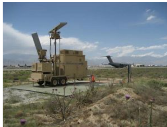
MERLIN SS200m Aircraft Birdstrike Avoidance Radar system installation at Bagram Airfield, Afghanistan (May 2010). This is the 7 th MERLIN system purchased by the USAF and the 1 st to be deployed in an active war zone.
