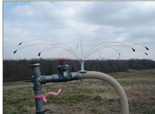
Figure 5: Bird spikes and other deterrents are used throughout the site to discourage perching of raptors.
